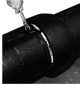
DISASSEMBLY OF 4"-12" FLEX-RING
