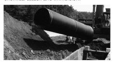
This 30" AMERICAN Ductile Iron Fastite joint treated-water transmission main was furnished and installed—as is most ductile iron pipe—with standard asphaltic coating approximately one mil thick on the outside.
